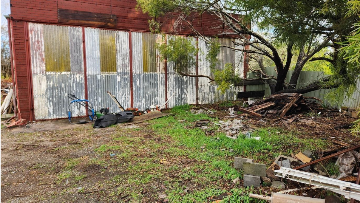
Photograph 7: North – west corner
