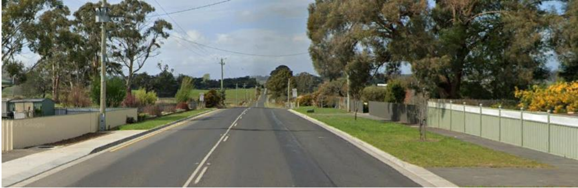
Photograph 7.2A – Available sight distance to the right
