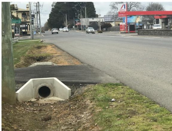
Figure 9 – Looking left along MVR from existing access
