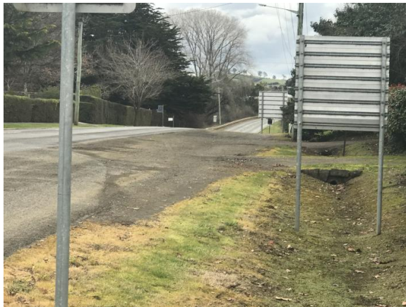
Figure 8 – Looking right along MVR from existing access
